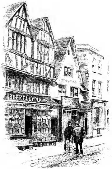
Old House, Tewkesbury.
